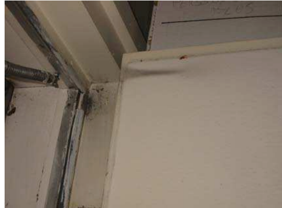
Figure 8: Laundry Room Door
